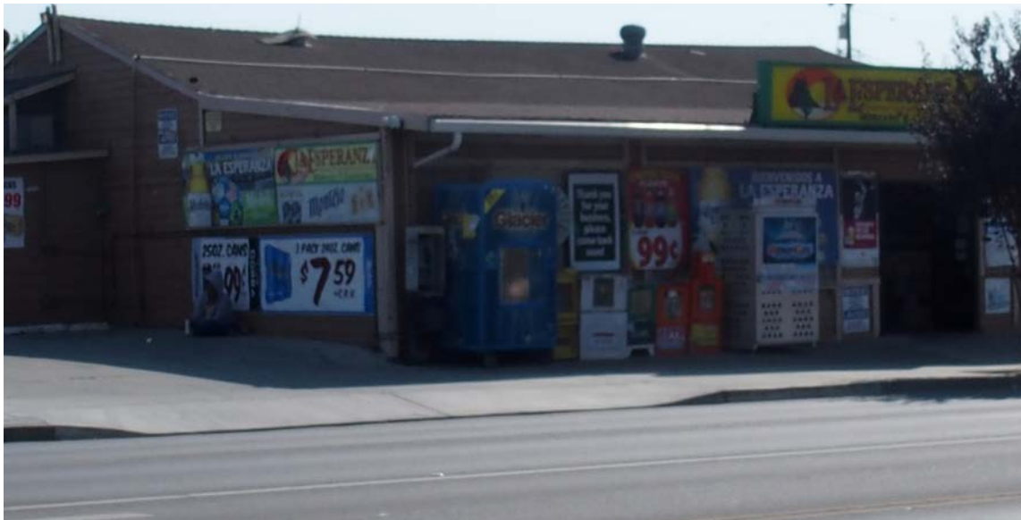
A lack of windows or posting over them with advertisements makes it hard to see into some stores.
